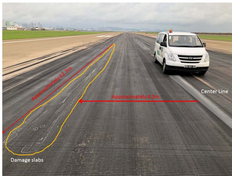
Figure 3: Runway slabs damage at Macau International Airport
